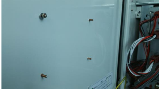
Figure 9 – 4 Fixed bolts (washers and nuts must be on every bolt)
